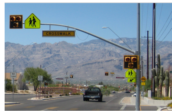
Level C: Pedestrian Hybrid Beacon/Signal
