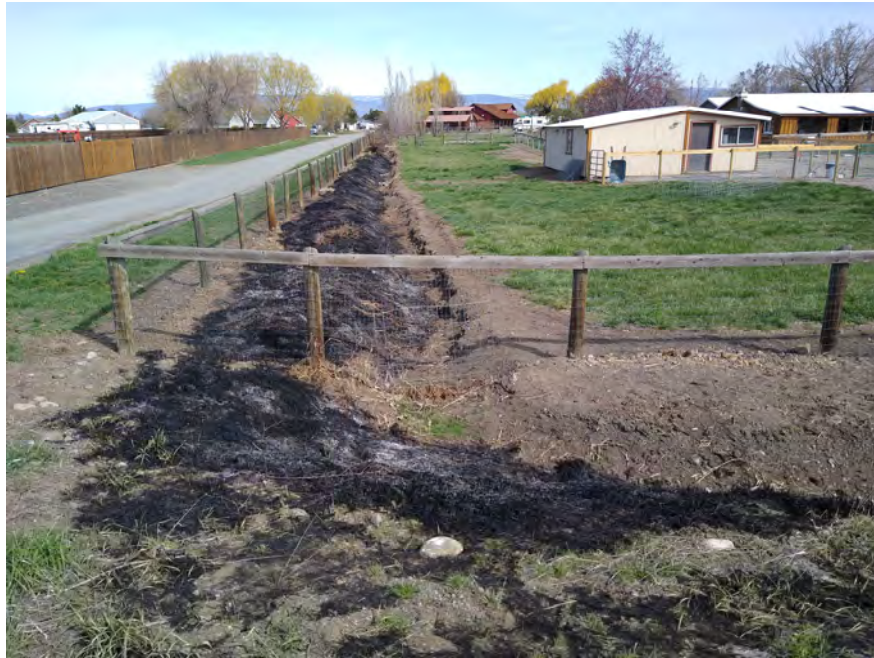
Photo 5. Typical irrigation ditch maintenance (“East Branch Lyle Ditch”) (view toward N, 4-7-2022). Note ash that would be captured during first flush.
