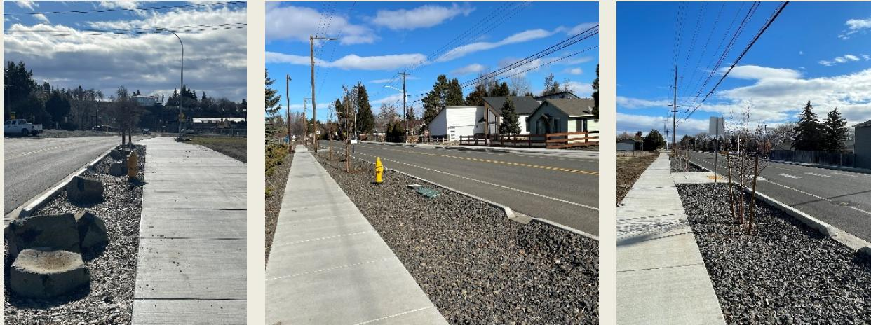
To ensure proper treatment, pre-treatment BMPs must be implemented to treat the first half-inch of rainfall. The Stormwater Management Manual for Eastern Washington provides options such as 60/40 bio-soil retention media, grassy strips, downturn elbows, and other BMPs, allowing design engineers to select the most appropriate solution for each site.
