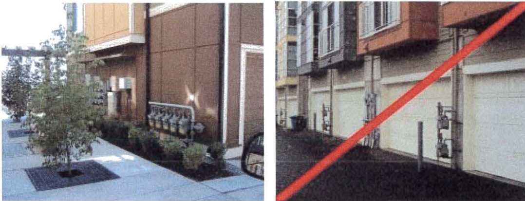
Figure 15.520.060(C). Good and bad utility meter configurations. The examples on the left are consolidated and somewhat screened by landscaping elements, whereas the right examples are exposed and degrade the character of these townhomes townhouses .
